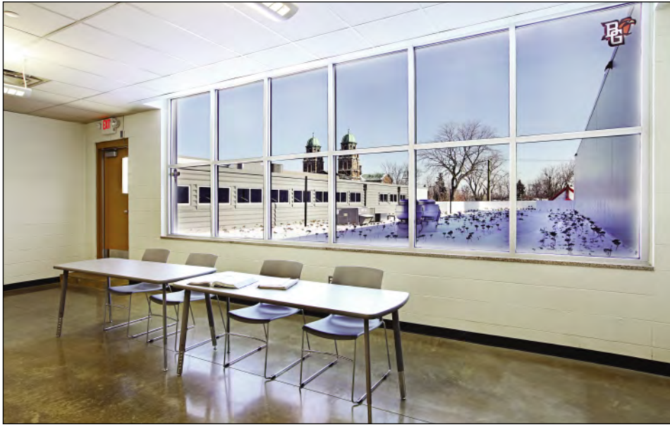
A 3,578-square-foot green roof, in the top photo covered in snow, helps reduce stormwater runoff while providing a learning experience for students.
